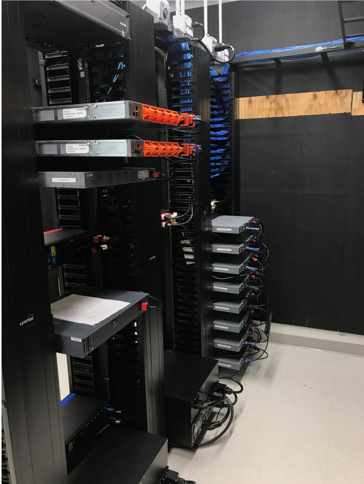
Typical Cable Management Photograph Example 003
