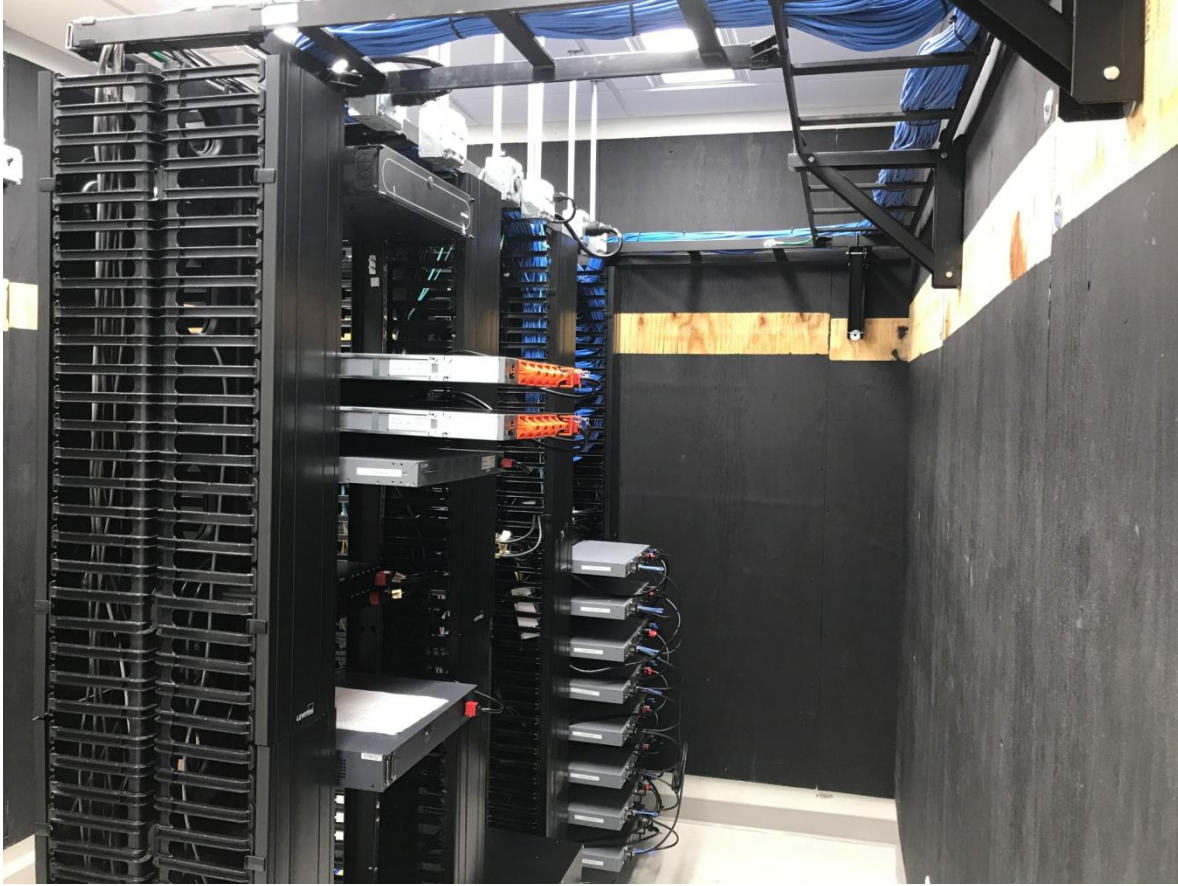
Typical Cable Management Photograph Example 005
