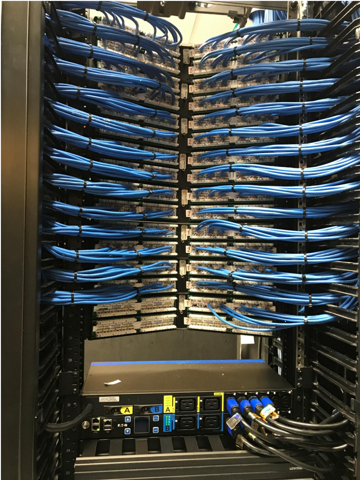
Typical Cable Management Photograph Example 004
