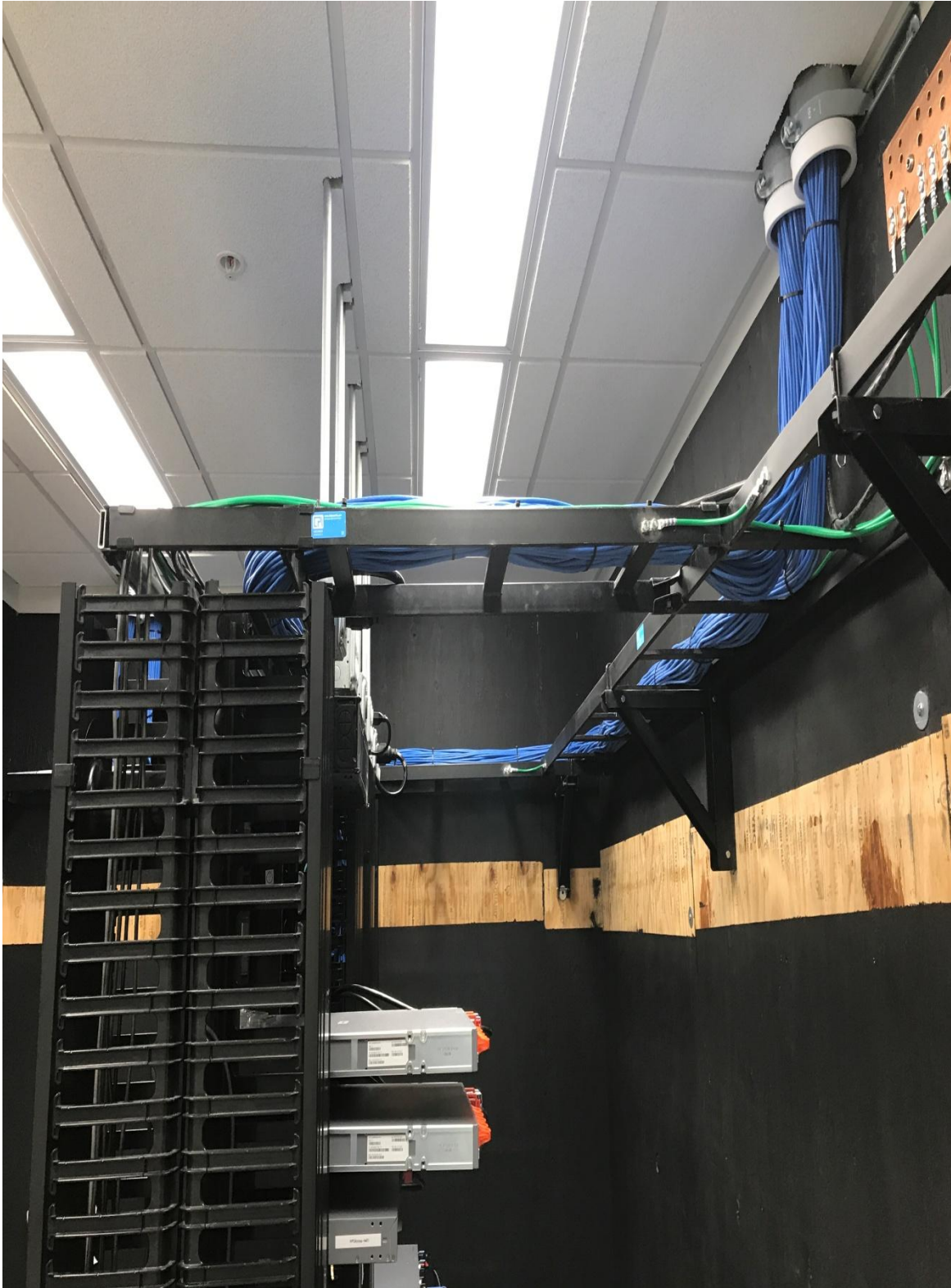
Typical Cable Management Photograph Example 001
