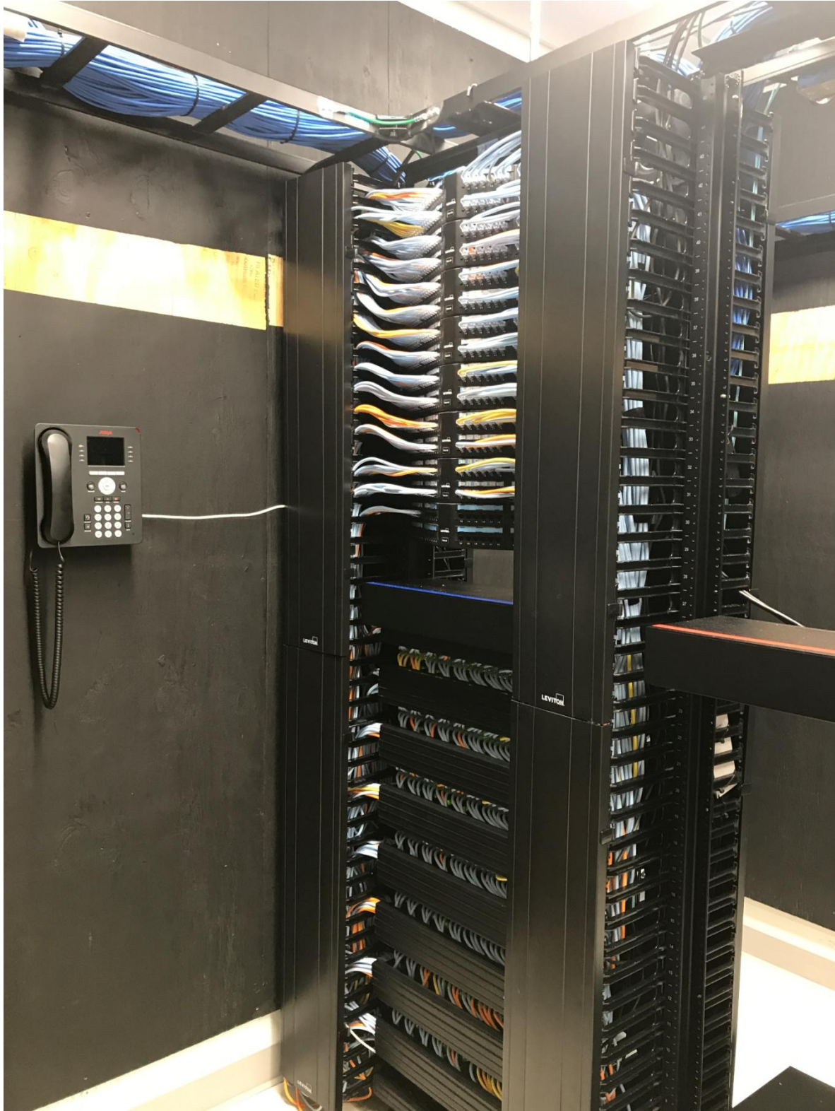
Typical Cable Management Photograph Example 002
